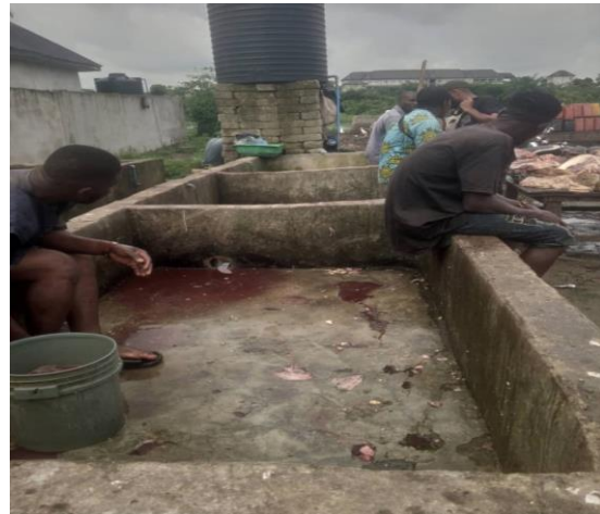
Figure V: Improved Trippery and gutter
